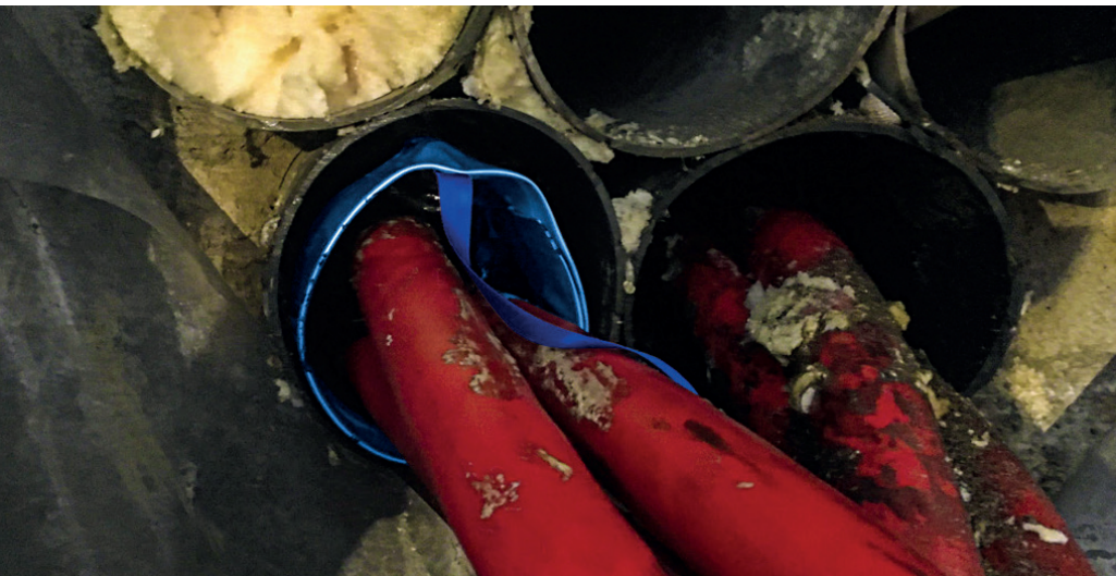
OKE installation with several power cables.
